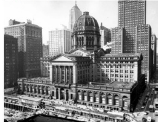
Chicago Federal Building lost 1965
