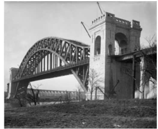
A view of the recently completed Hell Gate Bridge, circa 1916. Photo by the Detroit Publishing Company.
